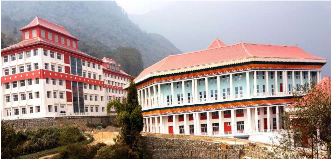
University Campus at Yangang, South Sikkim
