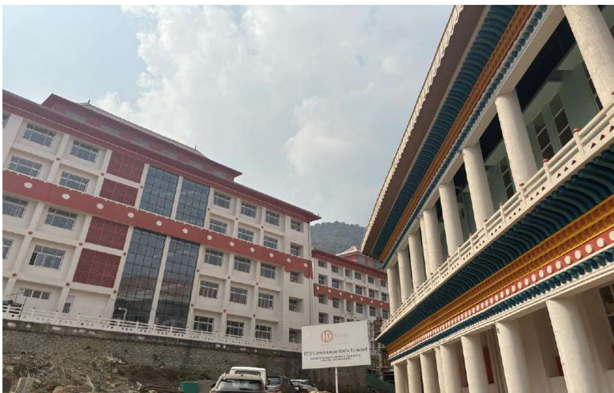
University Campus under construction at Yangang.
